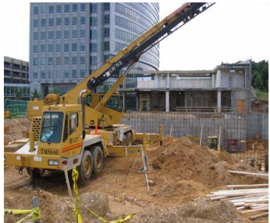
Figure 1. Crane on auditorium nose pulling formwork
