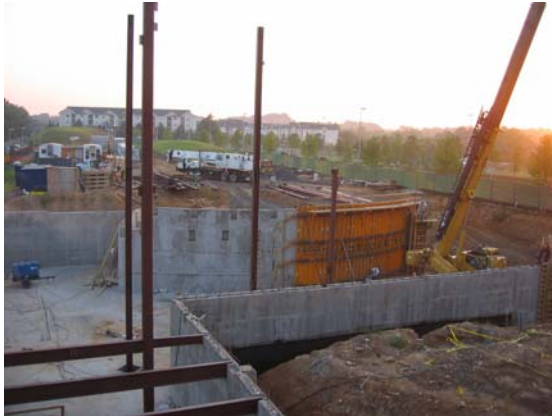
Figure 2. Steel crane setting up while concrete pulling forms
